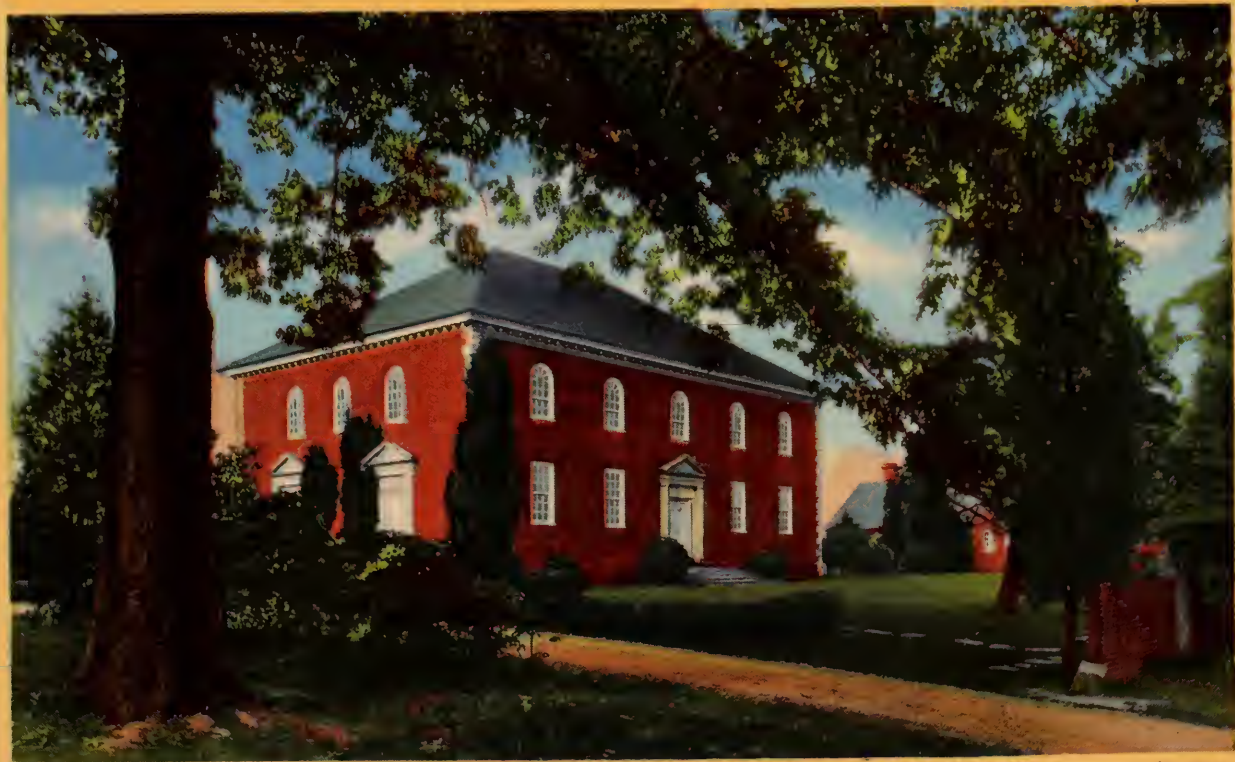
A-184—Old Pohick Church, Washington's Home Church, Built 1773, near Alexandria, Va.
